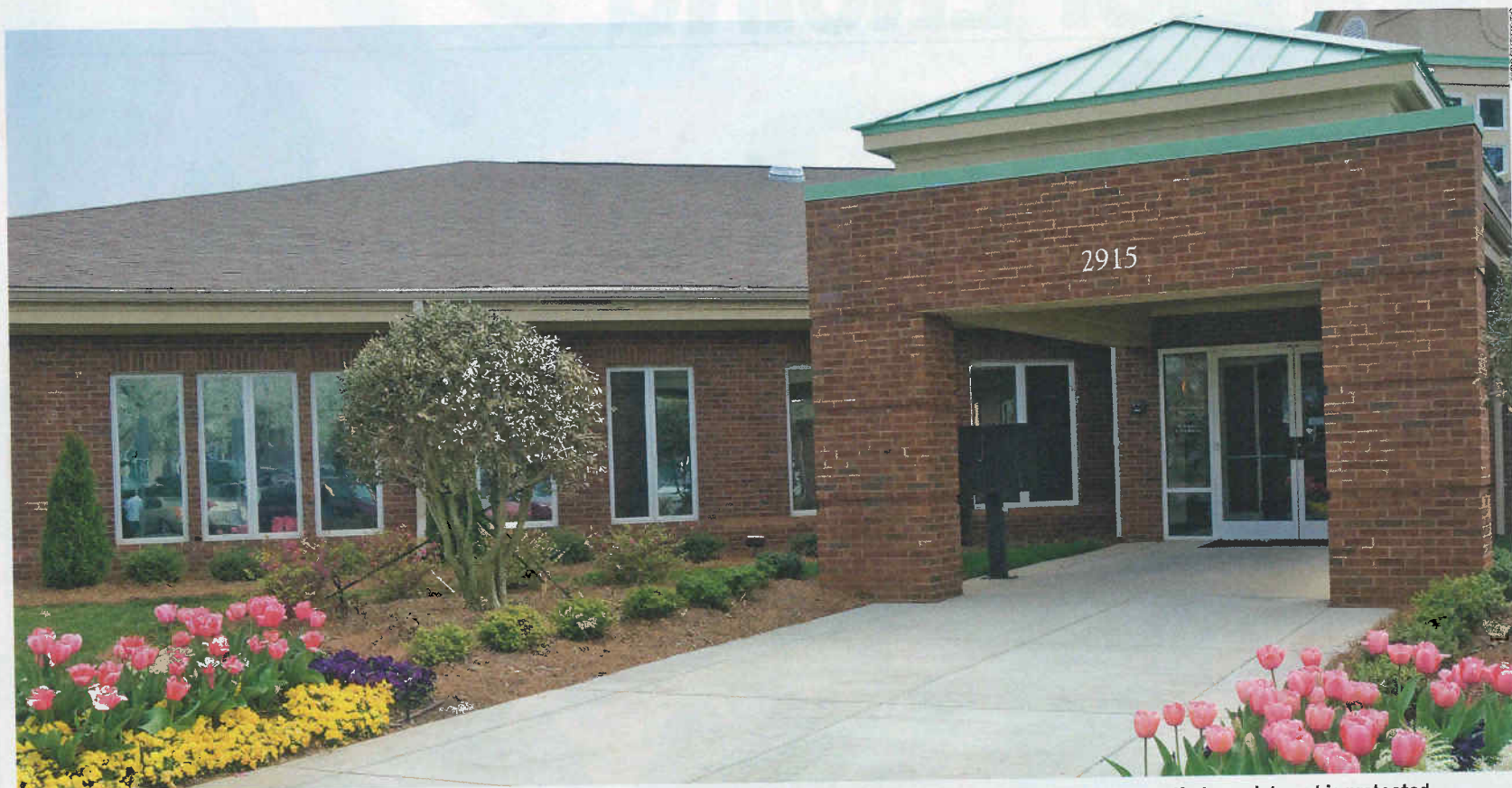
The surgery is likely to be one of the most valuable assets GPs own, both as an individual and a partnership, so it is important to ensure that your interest is protected
